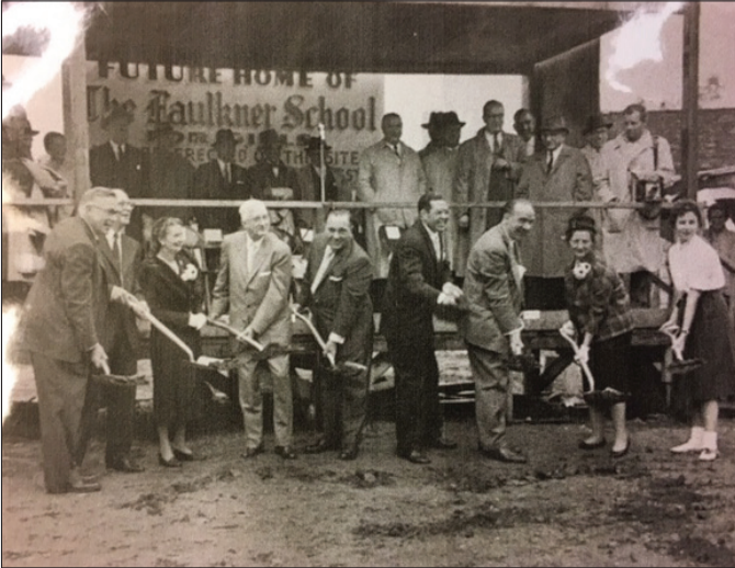
Groundbreaking for new school, 1958. Mayor Richard J. Daley, with spade in center; Principal Marion Davis at right in plaid jacket with spade.
