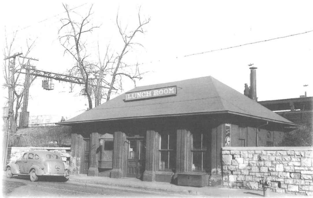
LUNCH ROOM AT 5529 S. LAKE PARK AVE. C. 1935
