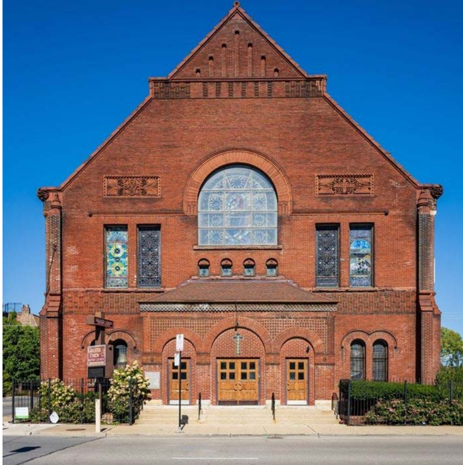
Greater Union Baptist Church, 1888, William Le Baron Jenney, 1956 W. Warren Blvd. Photo credit: Chicago DPD
